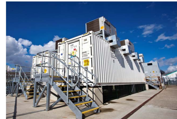
Customer-Led Network Revolution 2.5MW battery at Rise Carr
